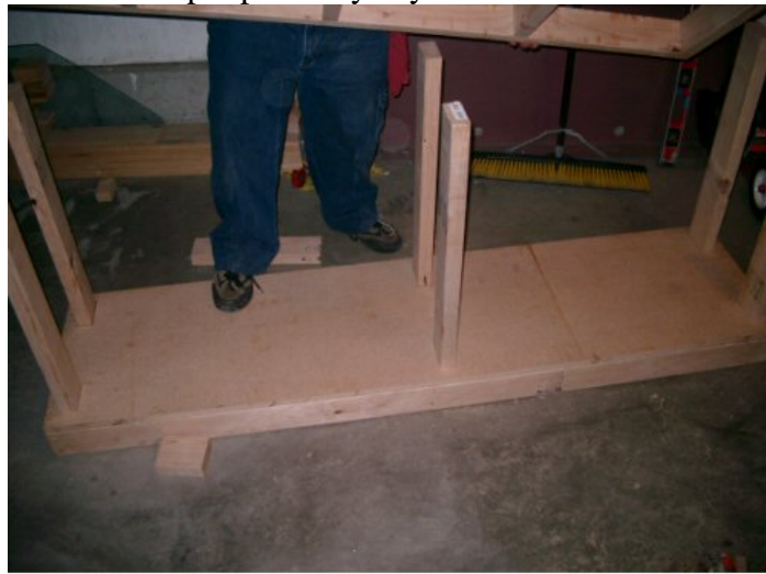
Construction of the stand
