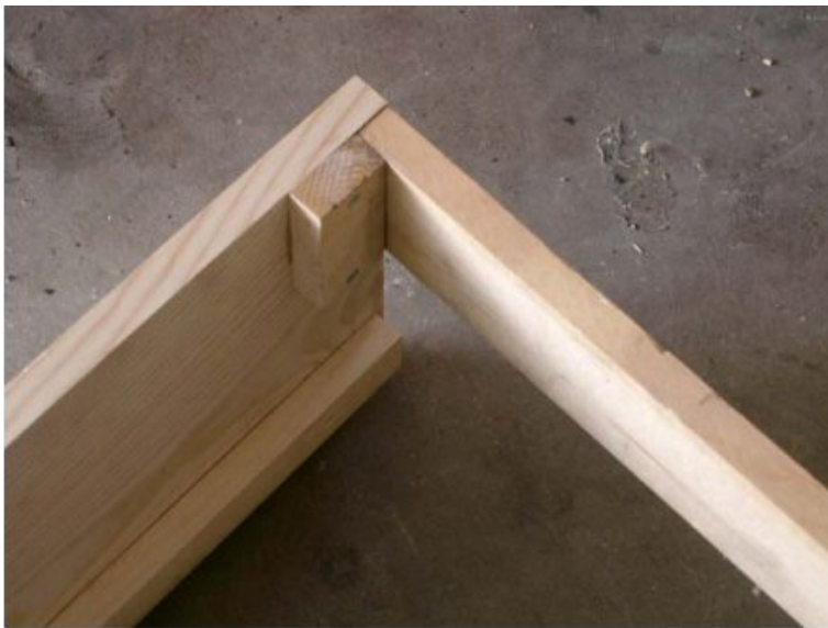
Building the canopy with cheap shelving wood
