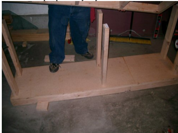
Construction of the stand
